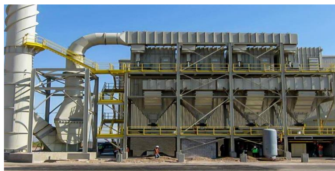
Figure 25: Industrial baghouse filter [IAC]
